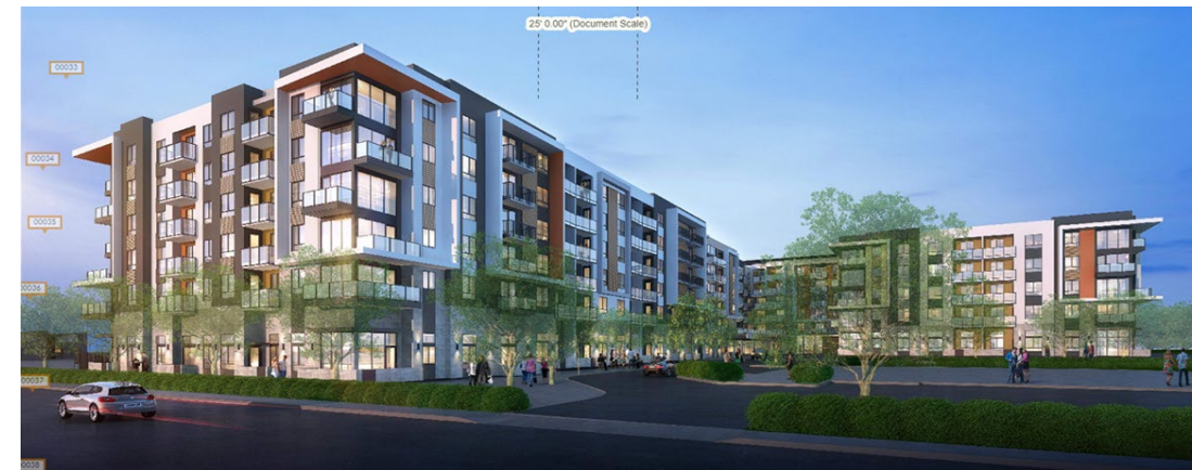
Convoy Square Development Under Construction
