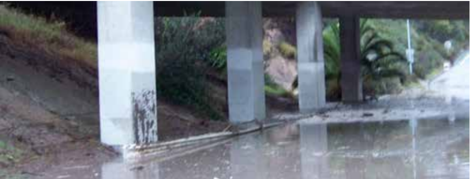
Flooded underpass on Aldine Drive
