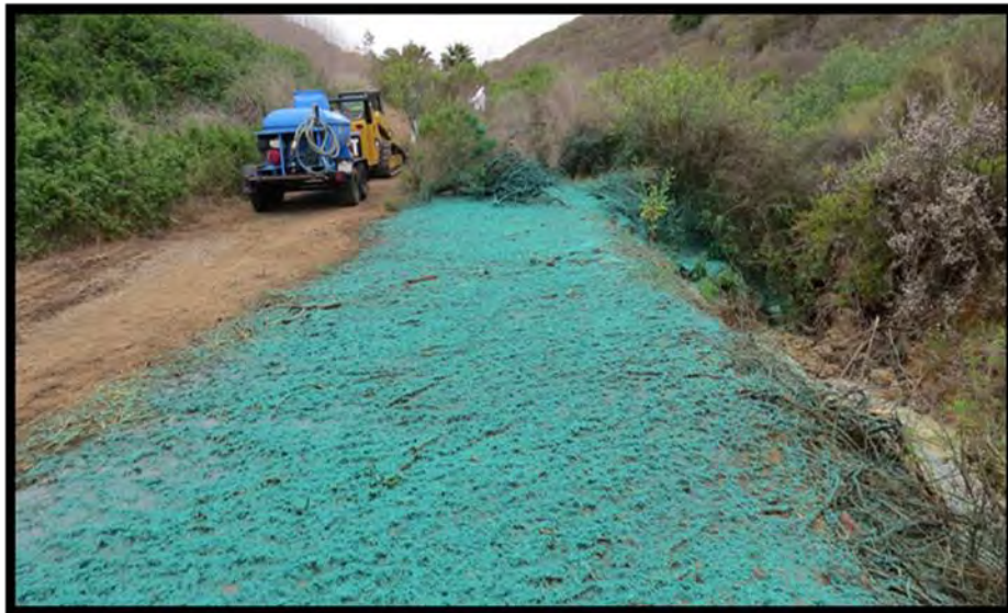
Stevenson Canyon Emergency Pipe Protection Restoration (Hydroseeding)
