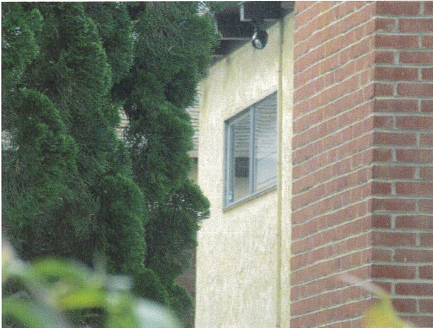
Photo 3: Detail photo showing the aluminum replacement window.
