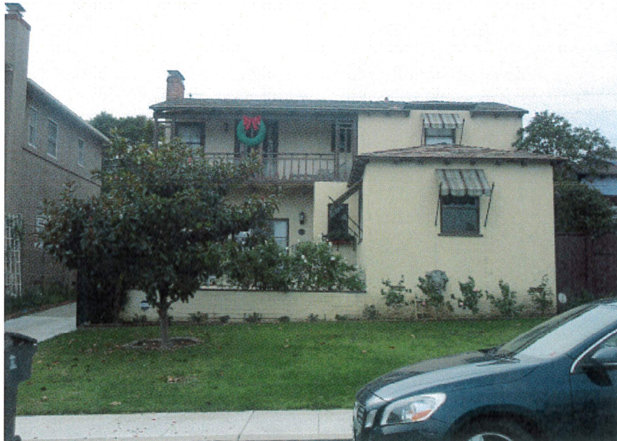
Photo 1: Looking southwest at the primary facade.
