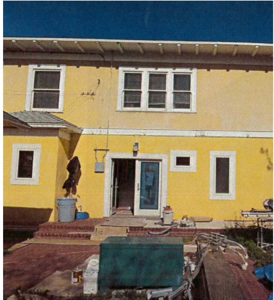
Rear After Unpermitted Alteration
