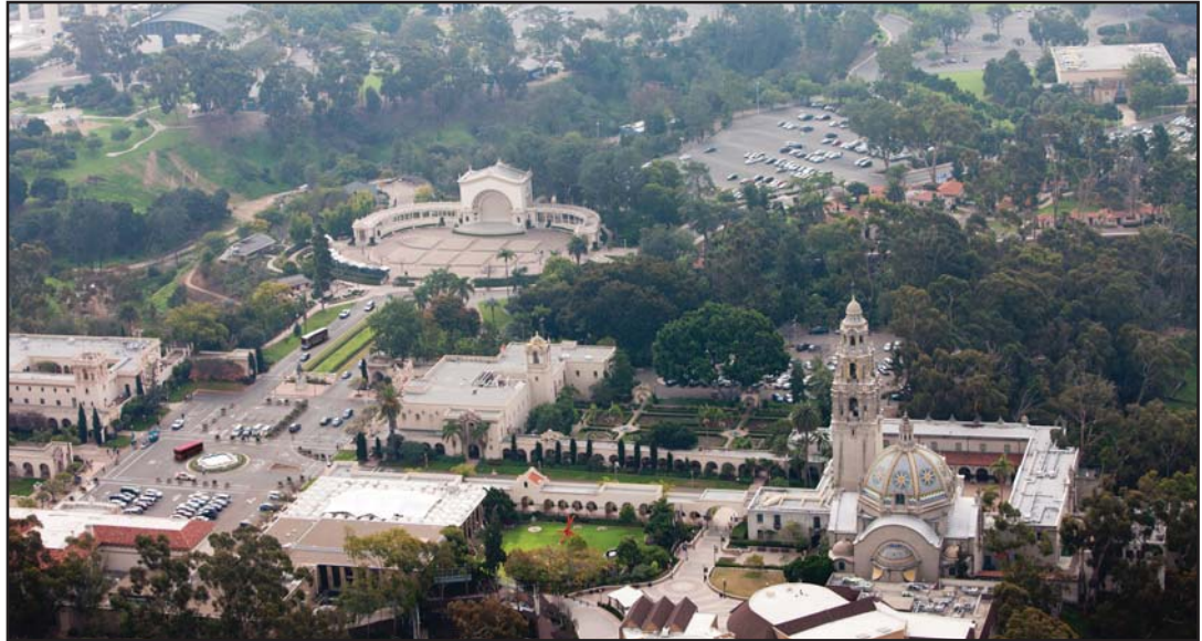
Existing Parking Lot from North
