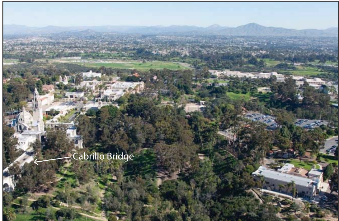
View of Cabrillo Bridge without Centennial Bridge
